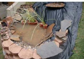
After digging and leveling; put the liner, dishes, and pump in place and do a practice run to see how the water flows. As you add the gravel the flow will change, so you can adjust as you need to.
